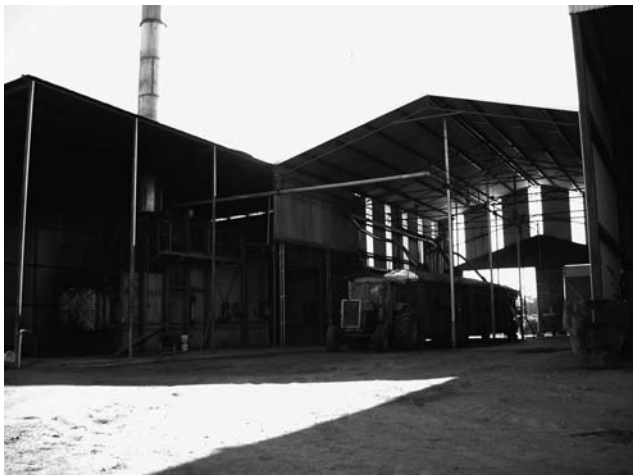
FIGURE 4.22 Distillation plant with container technique.
